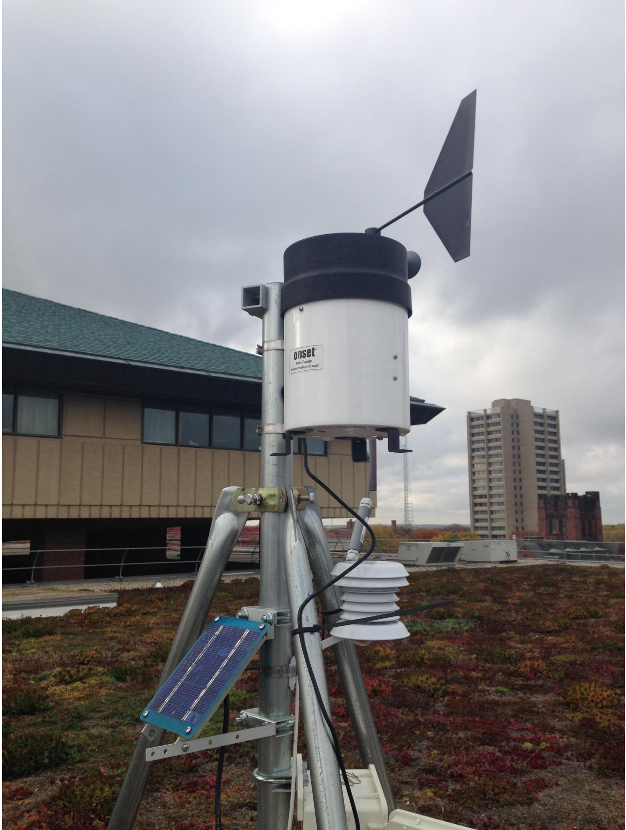
Figure 17. Weather Station on the east green roof.
