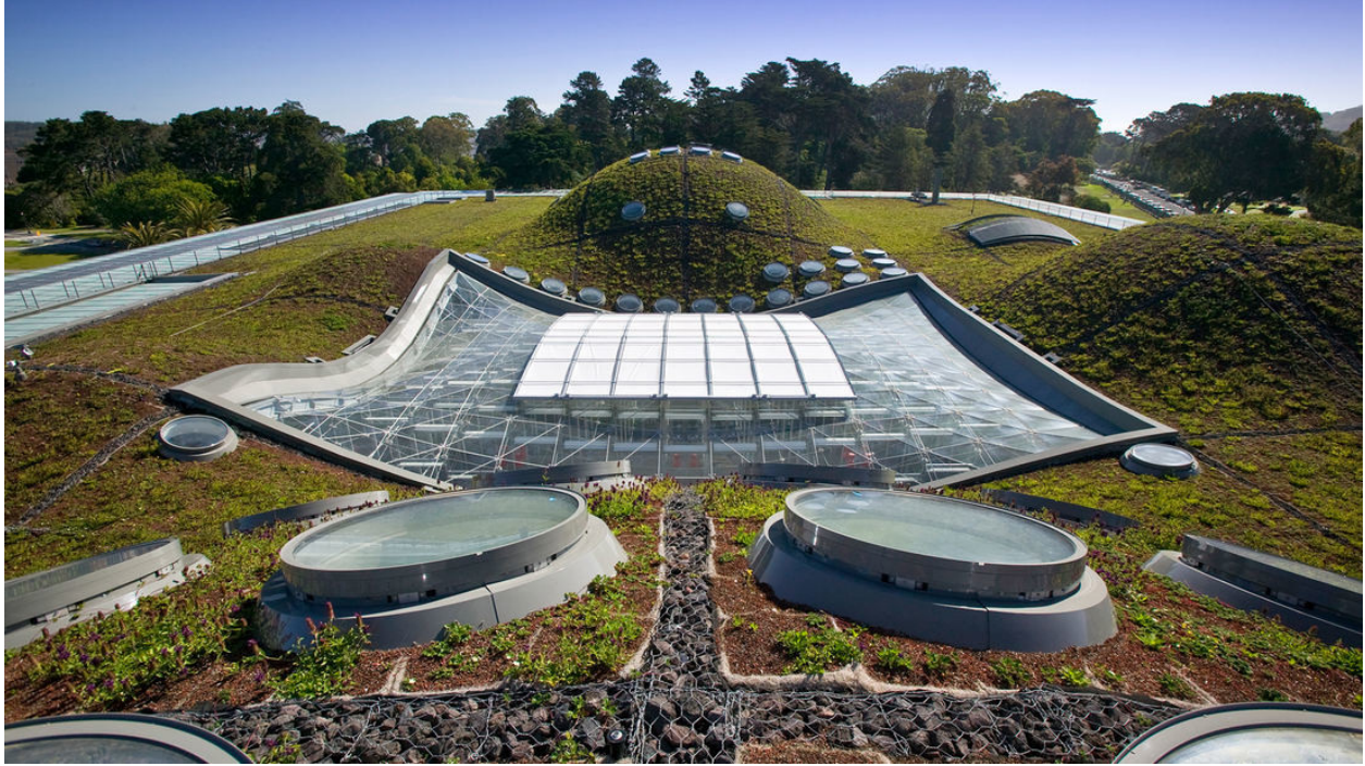
Figure 10. The skylight of California Academy of Sciences. Source:
